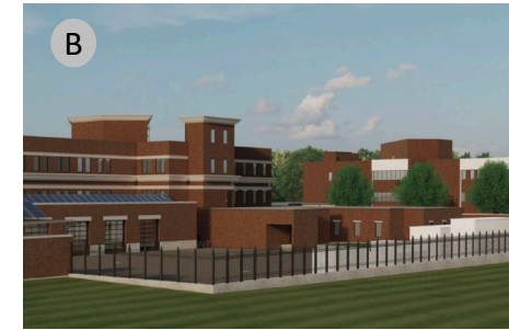
Power distribution and charging research area in 1 st floor west wing (AC/DC/Solar)
